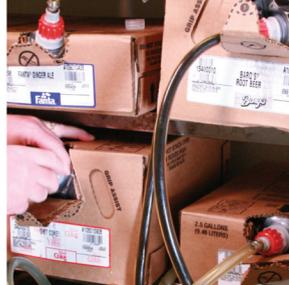
**Step 2.** Unscrew the syrup line connector and remove the empty box.
